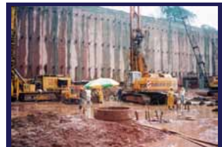
Exposed Wall Constructed under KB Slurry
