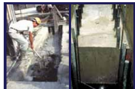
Concrete Rise Under Bentonite vs. KB Slurry on same project in Marine Clay
