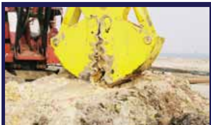
Excavating a Diaphragm Wall in Shore line Sands with Seawater Saturation and Tidal Influence
